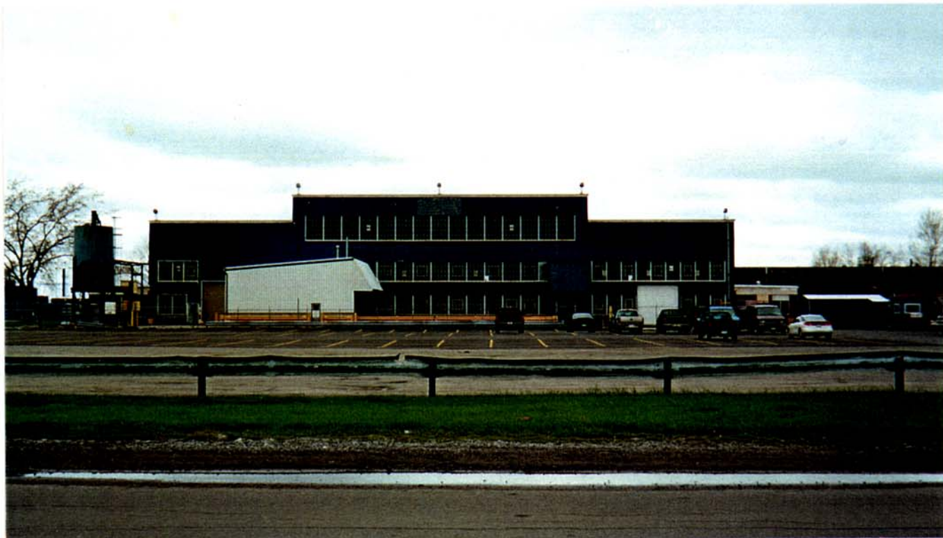
Photo 4. South elevation of Plant No. 5, facing north from Vulcan Street.
