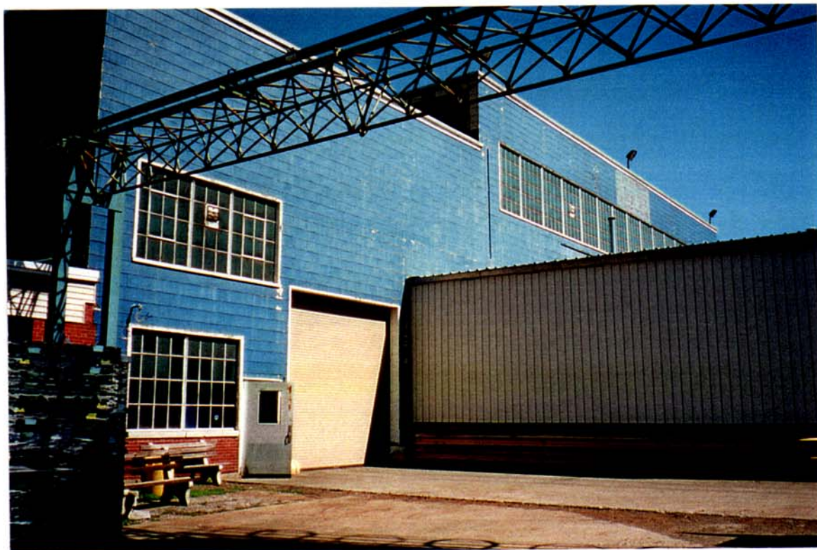
Photo 5. Detail of west bay, south elevation. Facing northeast.
